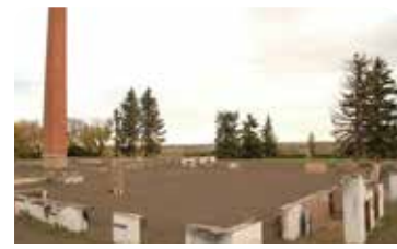
Stabilized ruins of the 2003 fire. Government of Saskatchewan, Photo by Calvin Fehr, 2004
